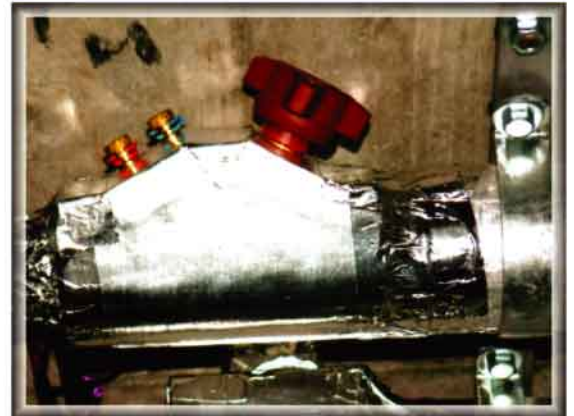
Preformed Valve Insulation Box
