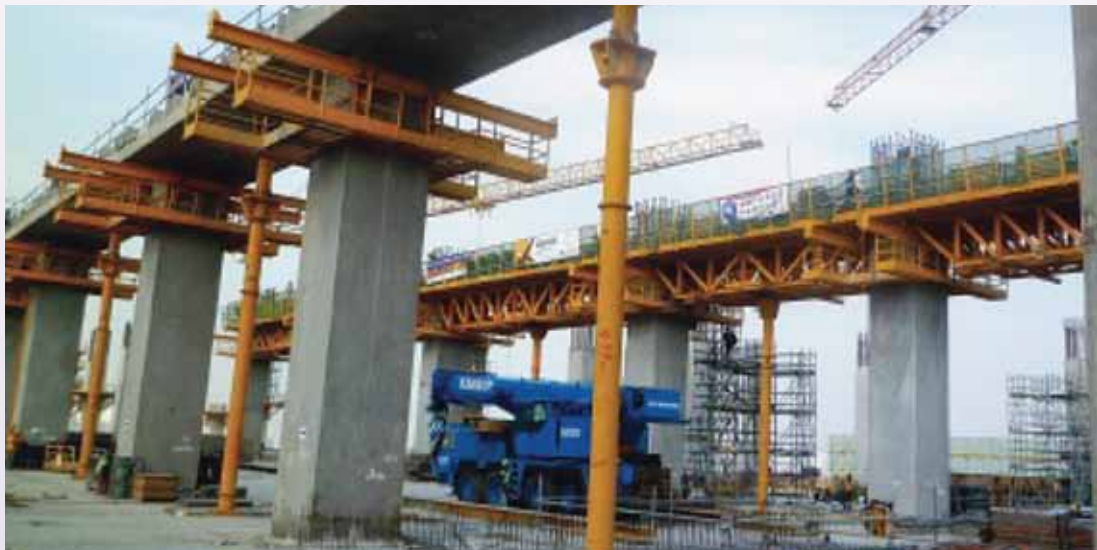
The use of Cordless tools enhances safety & productivity by eliminating wires from construction sites.
