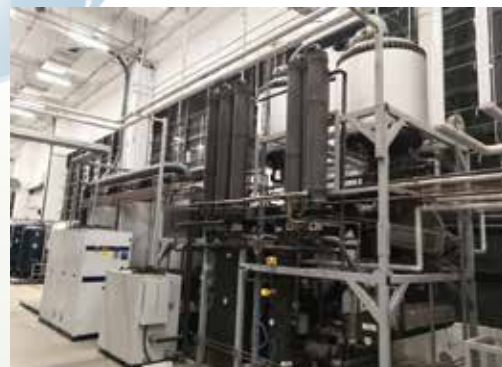
Activated Carbon System for Separation of Blowing Agents
