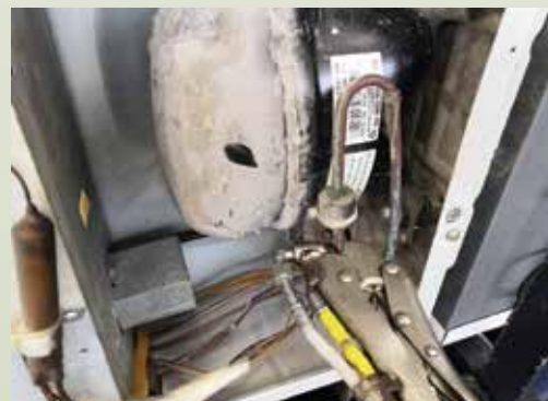
A Suction Plier Applied to the Refrigerant Circuit of a Refrigerator
