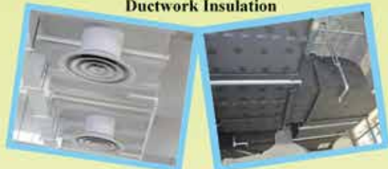
Duct Support Insulation (DSI)
