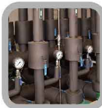
Prefabricated Armaflex On Elbow
