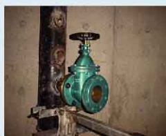
TEE-OFF DONE, READY FOR PIPEWORK CONNECTION.
