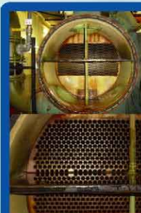
Clean tubes after 18 months operation
